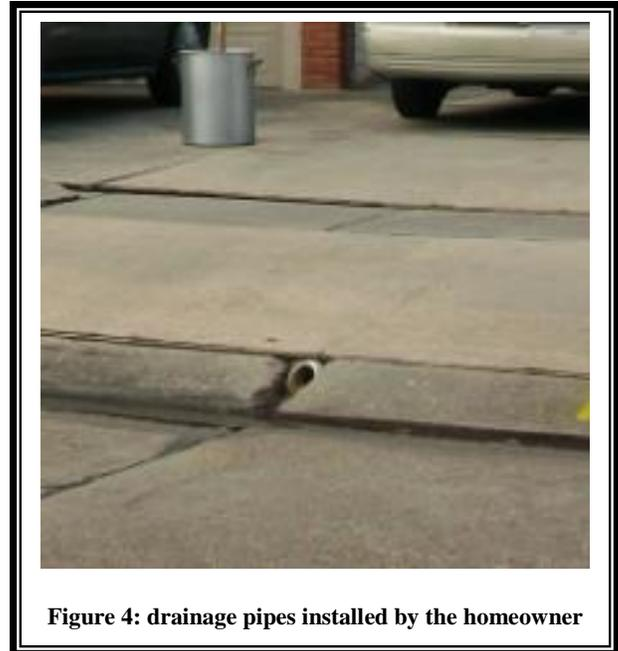
Figure 4: drainage pipes installed by the homeowner
